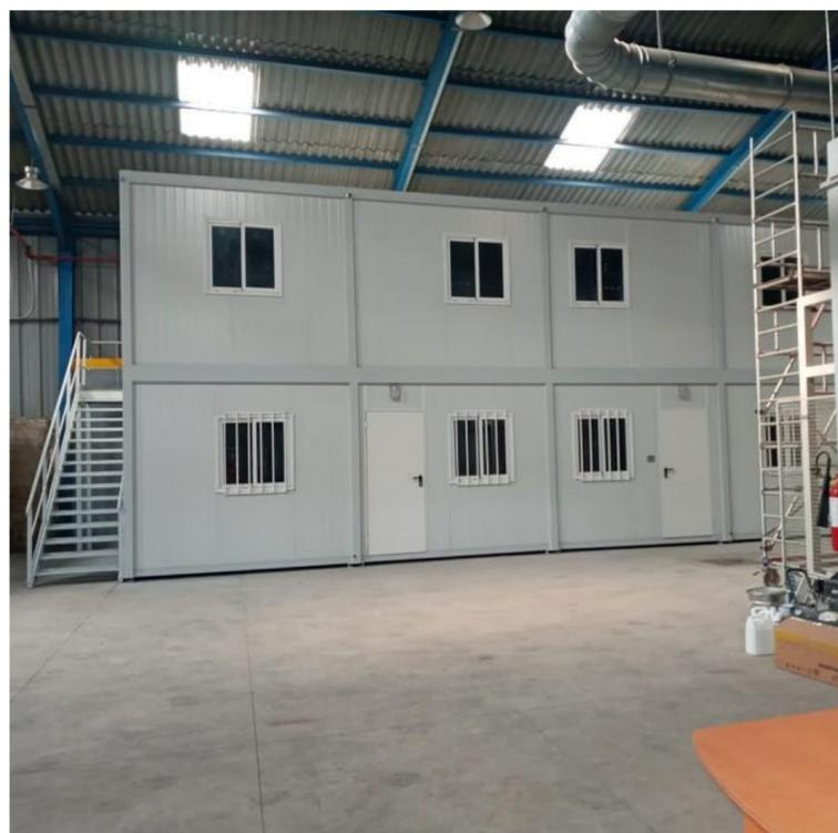
The galvanised steel structure, roof and floor ensure long-term durability, minimising maintenance costs. Speed of execution was a priority, with a production time of just 20 days and an assembly time of 24 days.
